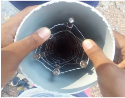
Figure 1. Reinforcement arranged inside PVC pipe
